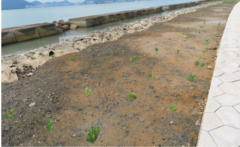
General View of Mangrove Eco-shoreline Upper Terrace
