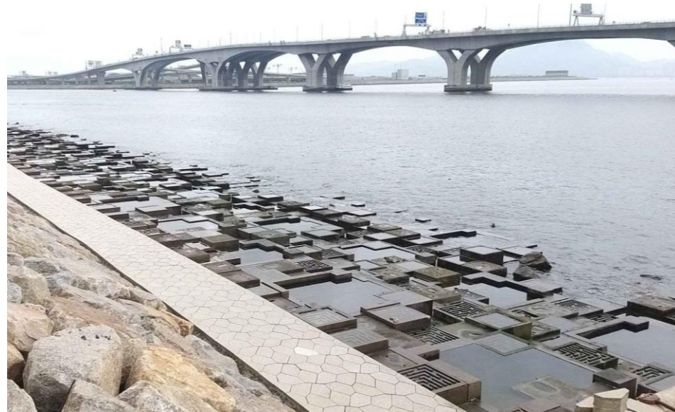
General View of Rocky Eco-shoreline
